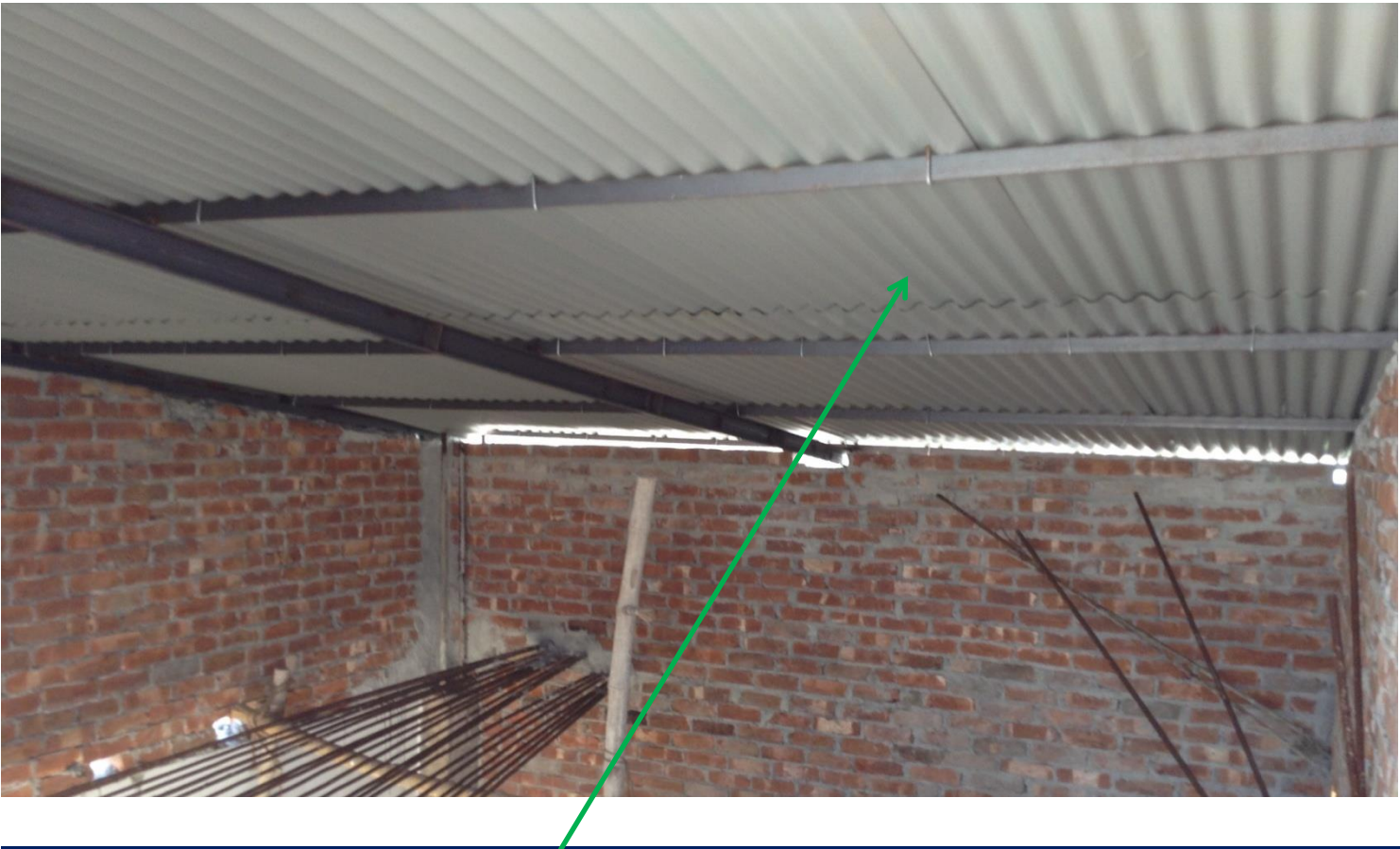
Temporary corrugated steel sheeted structure over stair
