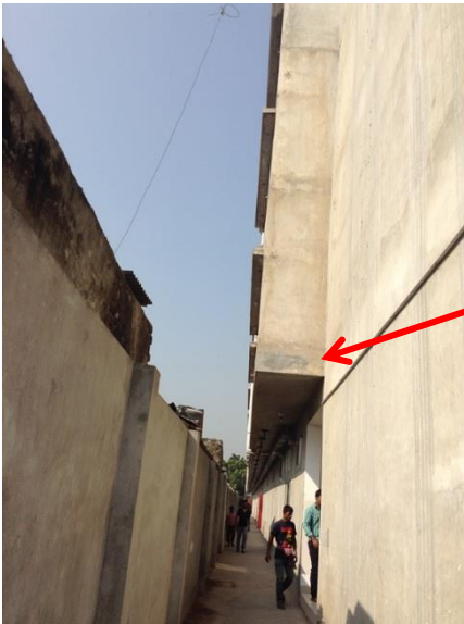
Permit drawing do not show cantilevers at north and south
