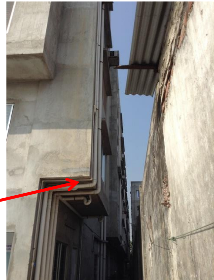
Permit drawing do not show cantilevers at north and south
