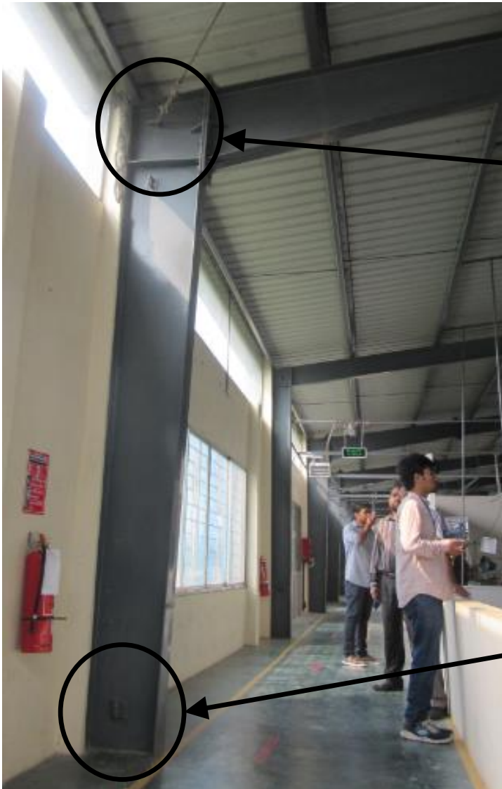
Connections for bracing unused
