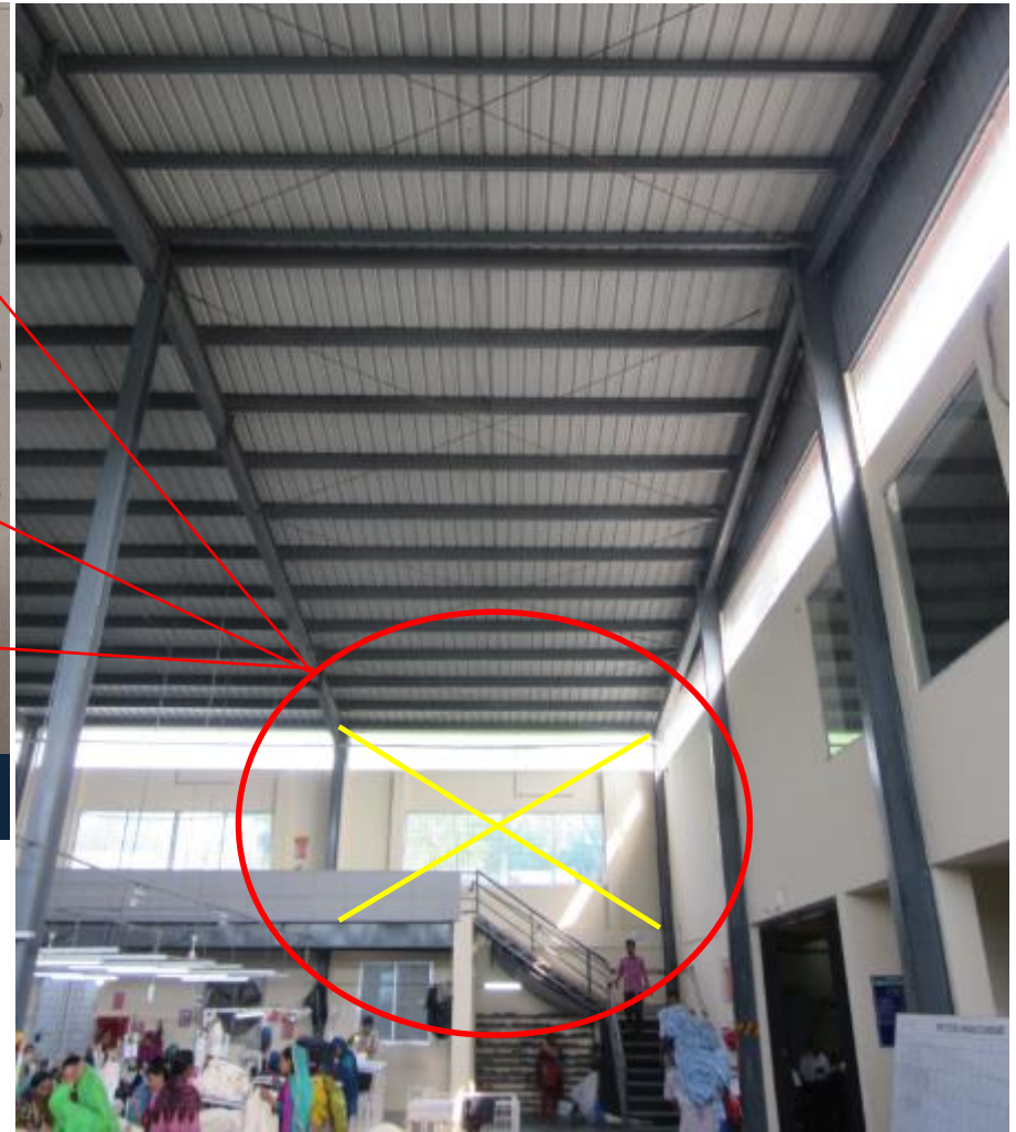
Lack of vertical bracing
